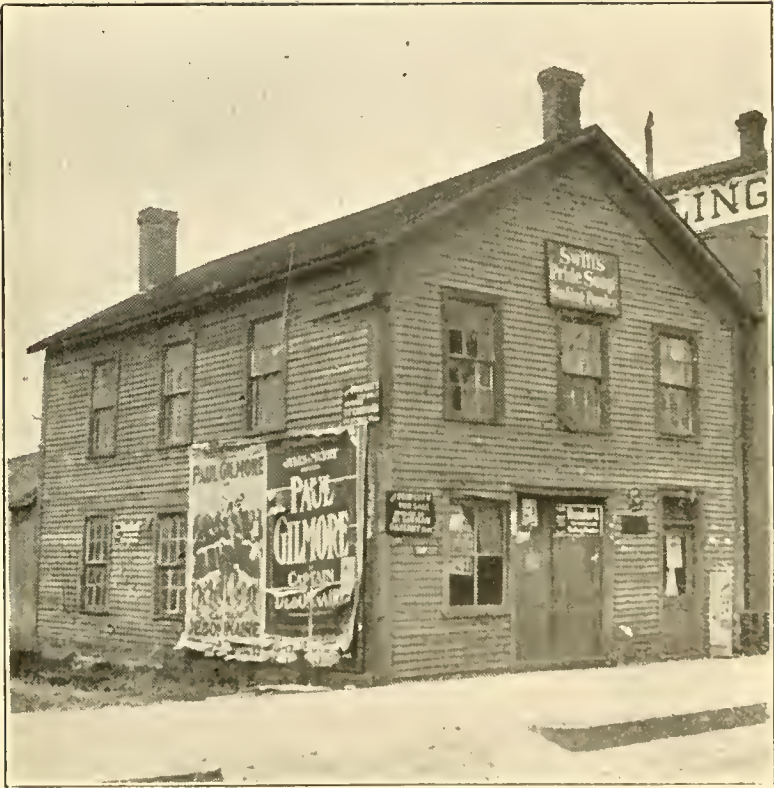
CRUMP HALL, FARIBAULT
